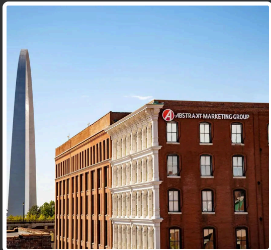
NORTH 1ST STREET
